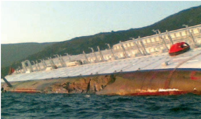
Figure 5 – Port side aperture at engine room location
